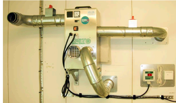
A DR-010B with DST humidistat EH4 controls moisture at a booster station
